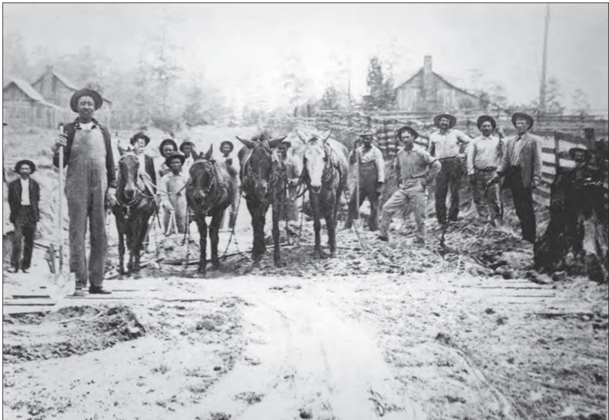
Figure 25 — Work crews attempted to maintain early roads under difficult conditions (courtesy Museum of West Louisiana).
