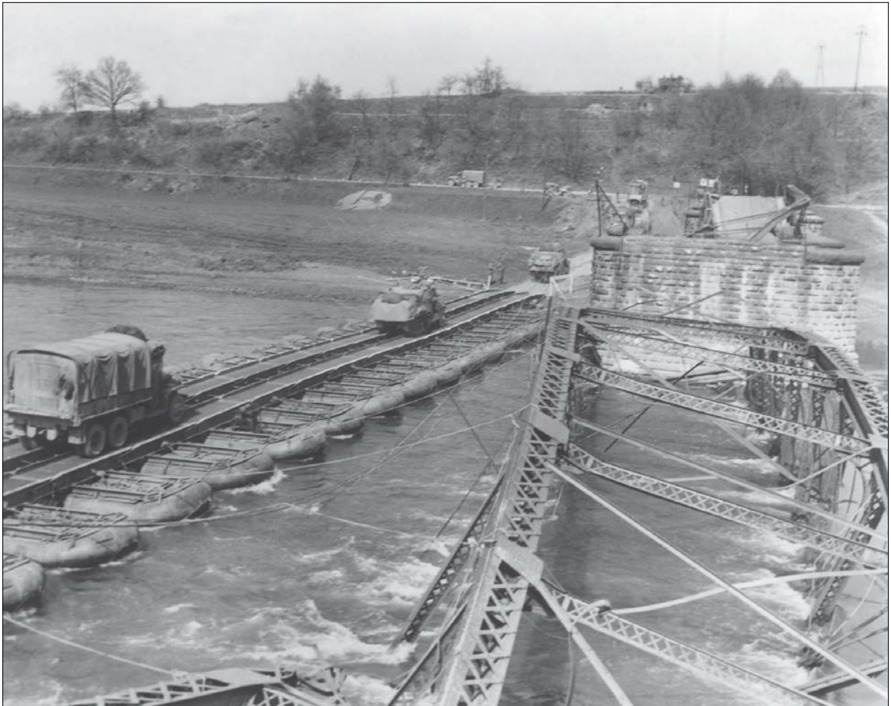
The 3rd Armored Division crosses a pontoon bridge spanning the Weser River at Eiselwerder, Germany. Engineers built the bridge next to an older span that had been bombed.
