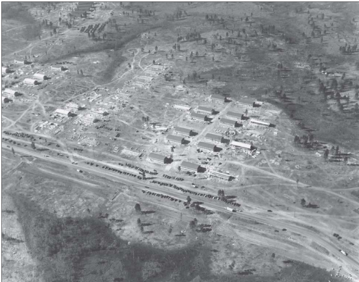
Aerial view of early Camp Polk construction in 1941.
