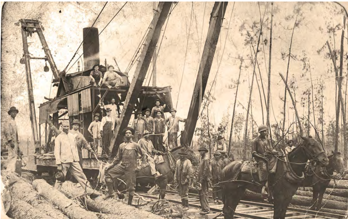
Figure 1-2.13. Steam skidder and crew loading logs in west Louisiana, undated. Logging crews were often racially mixed. Richardson (1983) reported that “Negro youth[s]” on mules were responsible for clamping the logs to heavy tongs at the end of the steam skidder cables. Source: On file at the Fort Polk Cultural Resources Office, Fort Polk, LA.
