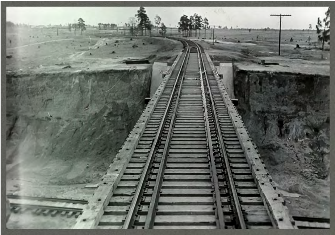
Figure 1-3.5. Railway connecting Camp Polk and Camp Claiborne in Vernon and Rapides Parishes, respectively, ca. 1942. Source: On file at the Fort Polk Cultural Resources Office, Fort Polk, LA..
