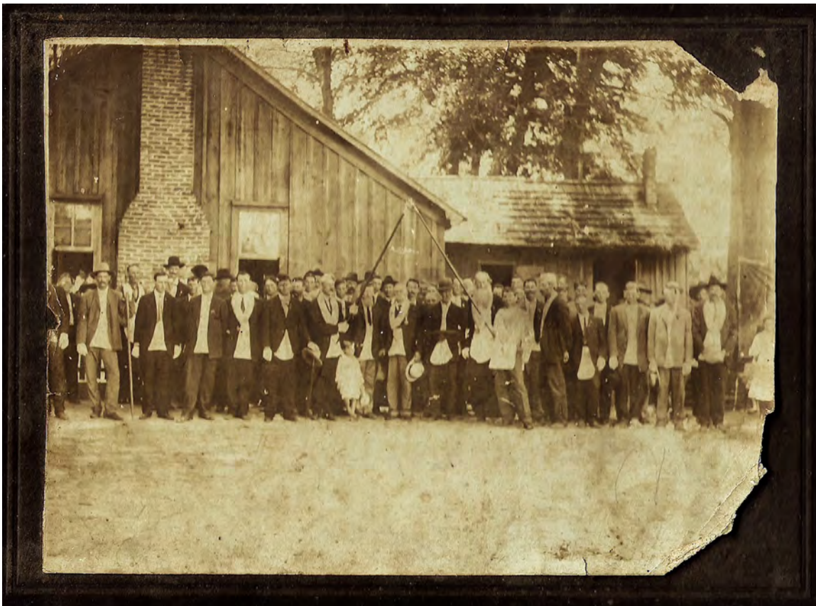
Figure 3-9.7. The Masonic Order on Peason Ridge sometime during the days of the Peavy-Wilson Lumber Mill (1917-1935). Source: On file at the Fort Polk Cultural Resources Office, Fort Polk, LA.
