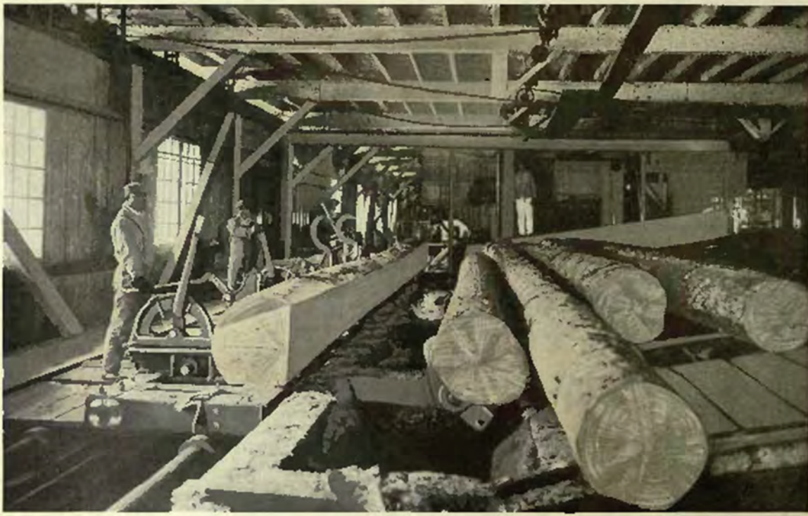
Figure 1-2.12. Large longleaf pine logs “ready to go onto the carriage and be converted into timbers suitable for heavy construction.” “The log carriage, which carried[d] the logs to the band saw, [was] a ponderous piece of mechanical equipment manned by a crew of four to six workmen. Source: The Long-Bell Lumber Company 1920 : 17-18.
