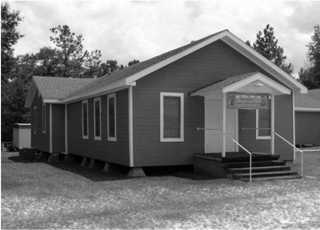
The original structure of the Sand Hill Church at its present location, now a part of the Oak Grove Baptist Church. The original church structure was rehabilitated and is resting on piers salvaged from the ruins of the Fullerton Mill. Source: Skip Cryer.
