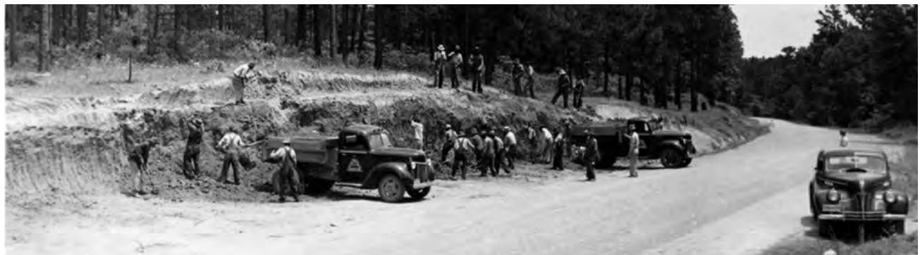
Figure 2-4.2. WPA road construction in the Kisatchie National Forest. Source: LOUISiana Digital Library .
